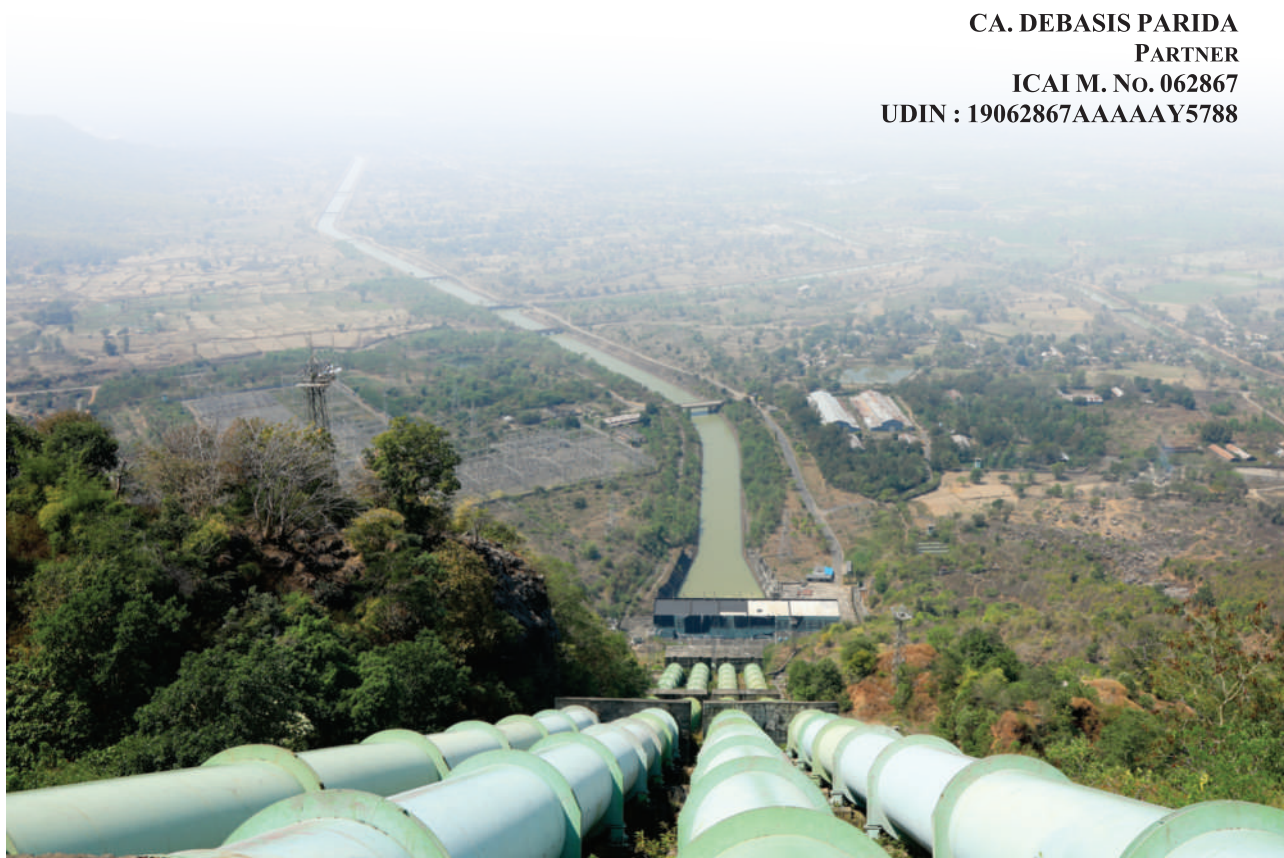
View of Water conductor system of UKHEP, Bariniput
